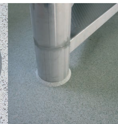
Triangle at installations without wall offsets
